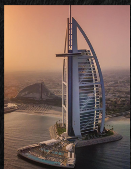
Burj al-Arab Abu Dhabi United Arab Emirates
